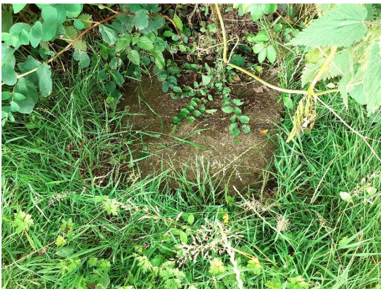
Existing highway drainage catchpit
